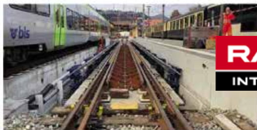
Gauge changers have been installed on two tracks at Zweisimmen.
