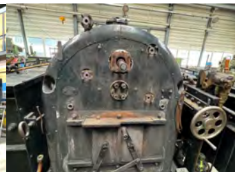
HG 3/4 Nr. 1 in Demontage
